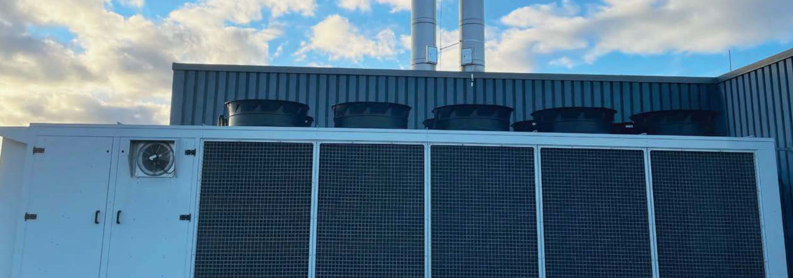
Image above: Refrigeration system for cooling processes in production (2021). Image to left: exhaust air scrubbing system with heat recovery
