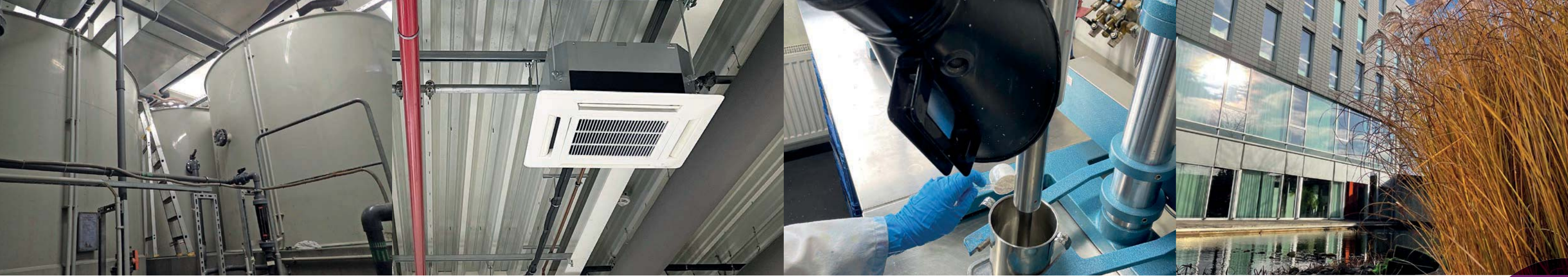
Images from left to right: collection tank for water treatment system, air conditioning for laboratory, air extraction system in laboratory, green outside space with pond
